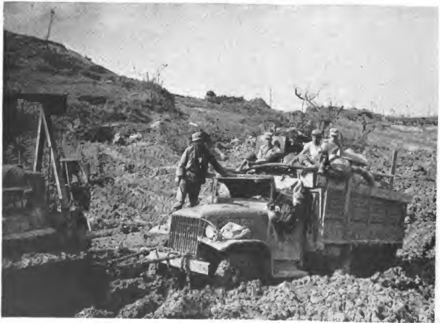
Top: A lineman exposes himself to enemy fire as he repairs telephone wires. Bottom: A bulldozer of the 302d Engineer Combat Battalion pulls a truck through a bad stretch of road north of Shuri.
